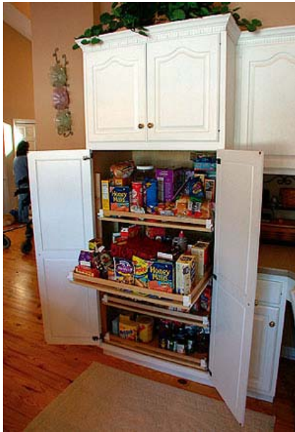
Pantry cabinet with knee space and easy-to-reach, full-extension shelves. Photos courtesy of PATH Partners
