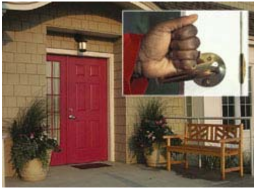
A no-step entrance with a side light and lever door handle adds accessibility.
