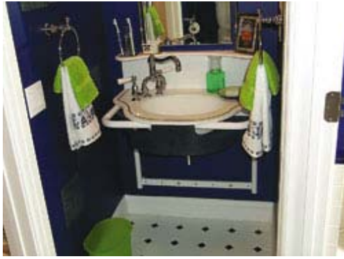
Universal bathroom cabinets can have "entertainment center" door hardware that opens to provide knee space (top). The adjustable-height lavatory (bottom) has knee space and easy-to-reach, lever-handled faucets.
